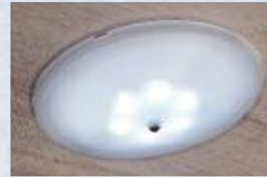
LED LIGHTING LED lights generate almost no heat compared to incandescent lights and use substantially less power.
