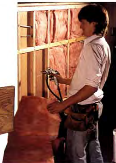
Insulation Cut & Glued Between Studs. Unlike blanket-laid insulation, Jayco's stays put; won't leave uninsulated spots; retains high insulation value year after year.
