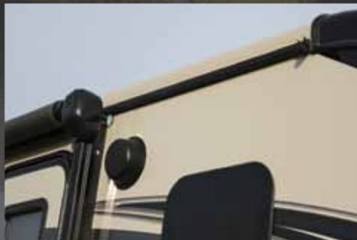
ROLLED ROOF EDGE PROMOTES INCREASED WATER RUNOFF
